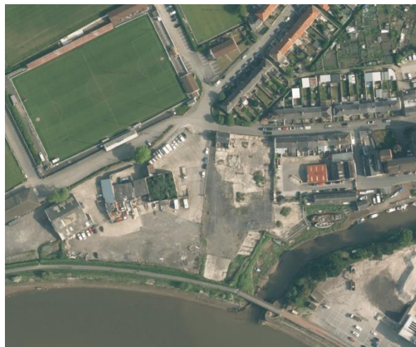
Aerial View of site
