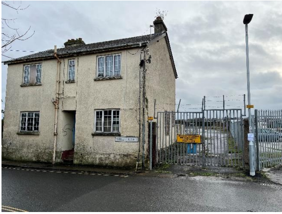
The site viewed from Mill Road
