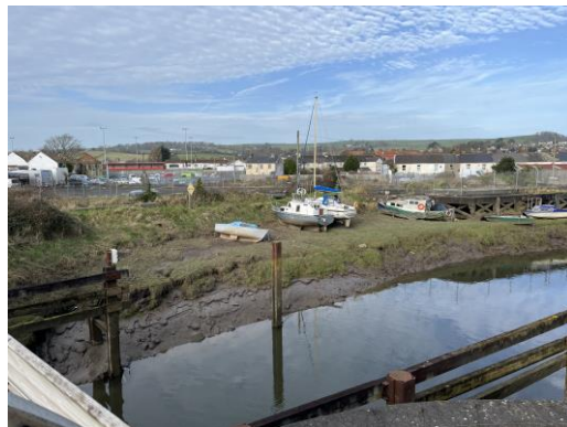
Site viewed from across the site from the (Tarka Trail)
